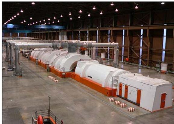
**Fig. 7: Steam Turbine at a Nuclear Facility**
