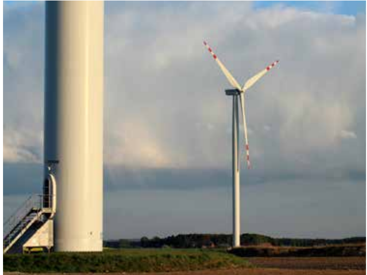
Figure 1 - Typical wind turbine environment
